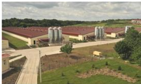
Photo of the grow-out farms for laying hens at Avis, July 2011
